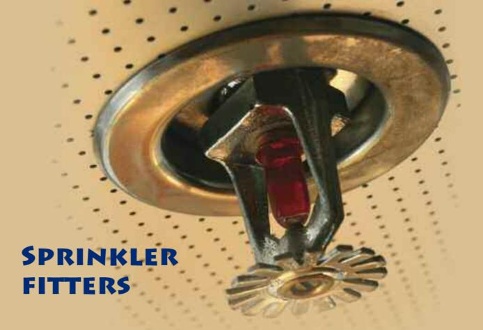
Sprinkler fitters literally save lives through their work. Sprinkler fitters are pipe fitters that specialize in the installation and maintenance of fire protection systems.
